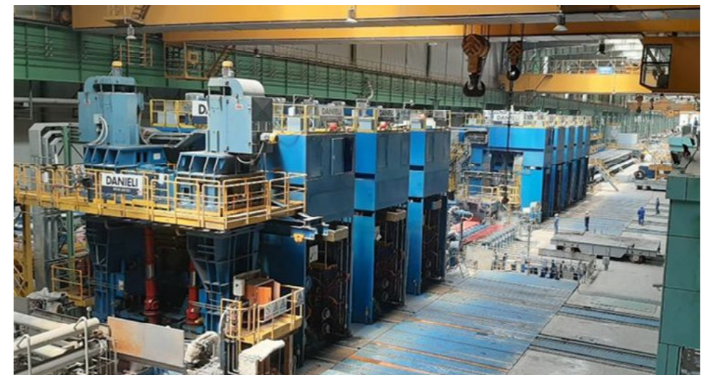
Figure 3: DUE® rolling mill at Shougang Jingtang (P.R.China)
