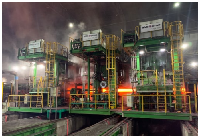
Figure 2: Reversing Tandem Mill with CCS-1500 Universal Mill Stands for rolling of jumbo beams (reference Nucor Yamato Steel, USA)
