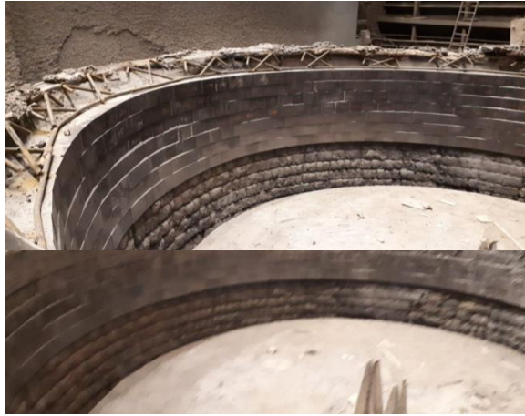
Figure 5. Shotcreting Castable before and just after application
