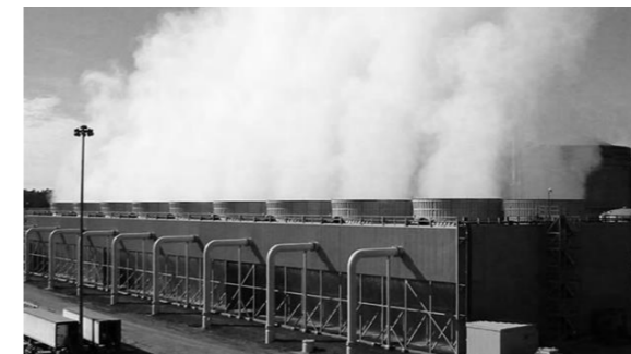
Figure 1. (Direct contact evaporative coolers) Wet coolers
