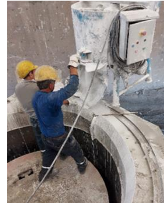
Figure 3. Free Flow Lip Castable Application
