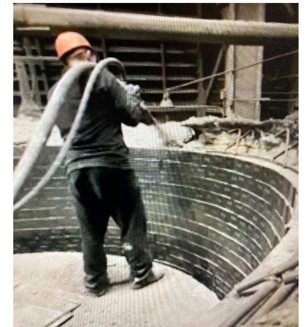
Figure 4. Shotcreting Castable Application
