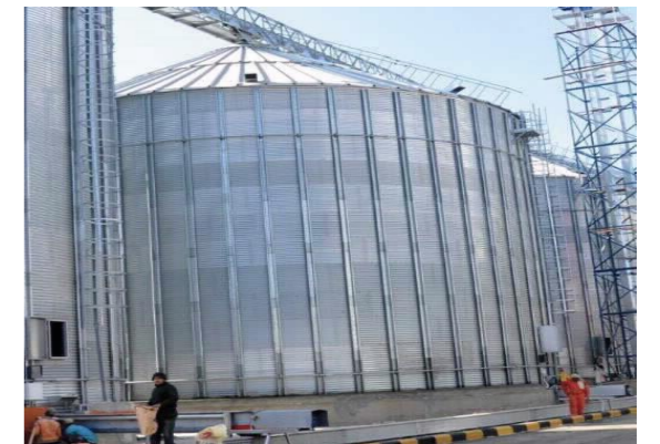
Fig. 1 Shows a silo which has dull and shiny parts on the body.
