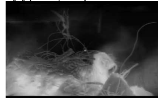
Figure 5. Scrap in the shaft preheater
