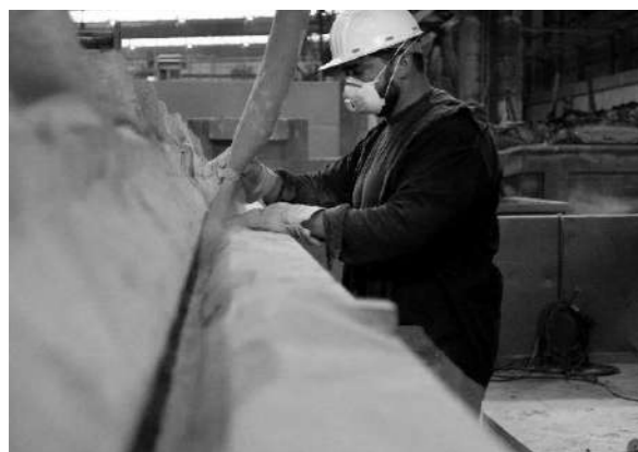
Fig. 2. Installation of a dry – mix.
