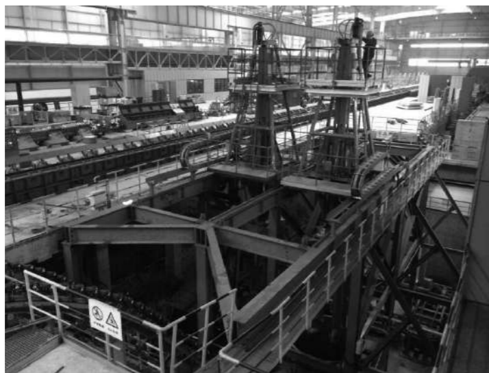
Figure 11 - Pouring Reel Outlet with Water Quenching Tanks
