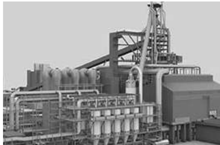
Figure 7:- 3D Model of the MERIM on the Blast Furnace.
