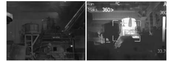
Figure 4: Real and thermal image of ladle
