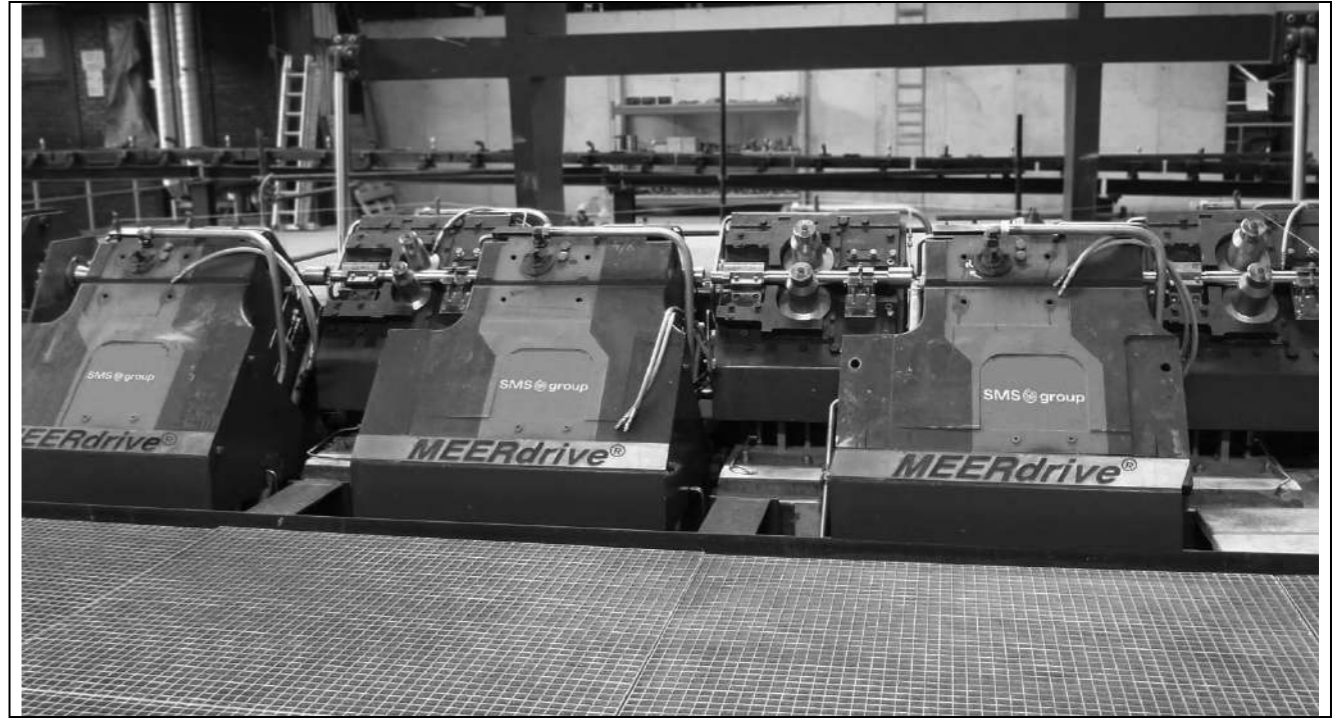
Figure 3: A recent MEERdrive® installation
