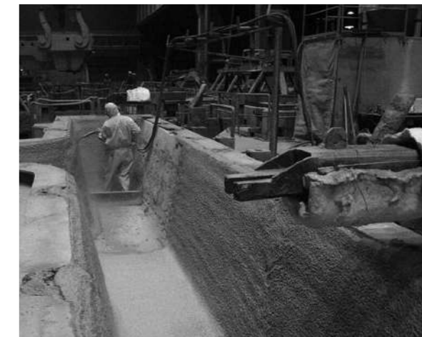
Fig. 1. Wet gunning of a tundish wear lining.
